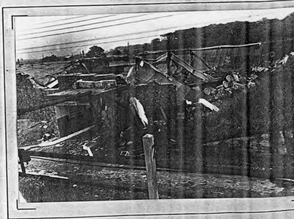
⑥ Further view from S.W. showing exit blocked.
