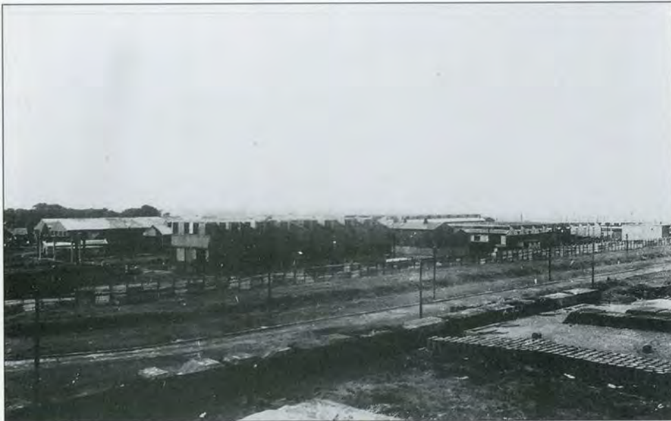
View from the observation post looking south west, October 1945. Lawrence Gale from Woolwich Arsenal was appointed Superintendent in July 1940, taking nine staff with him. The first shell came off the production line in September 1940. There were between 50 and 100 employees when it opened.
